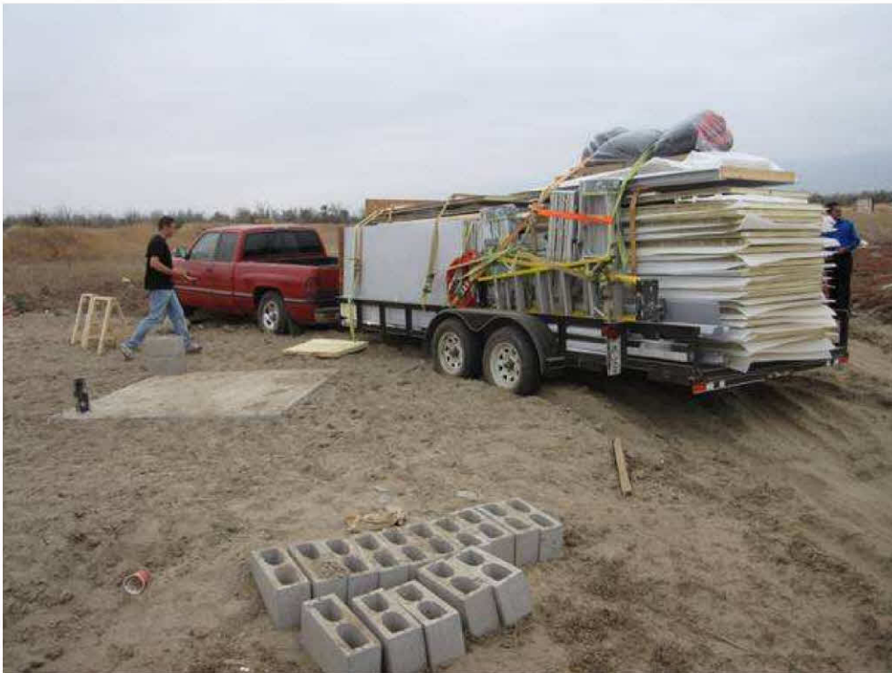
Trailer arriving at the build site fully loaded.
